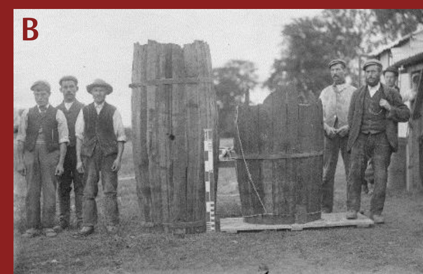
Excavators in 1897 with wooden barrels from wells in Insulae XVII and XVIII.
